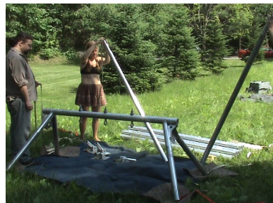
Feeding tensioning strap through next pair of leg sections.
