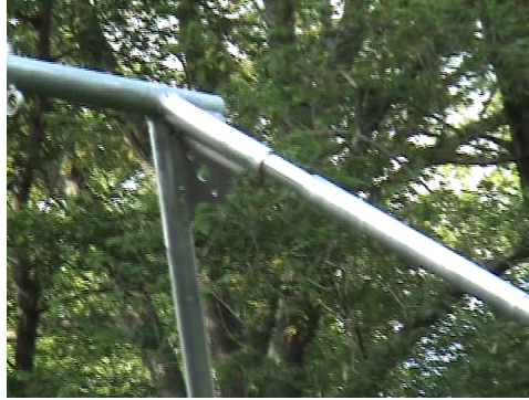
gap opening between top bar and pole. This one is large and should be shaken out before continuing.
